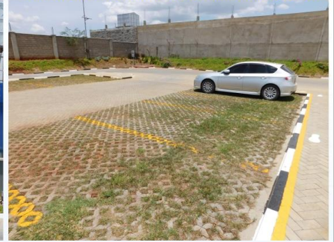
Lattice Pavers finish on Parking Lot
