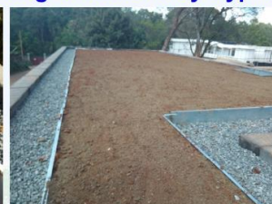
Preparation of Green Roof using Crushed Clay Byproducts and Planting Media
